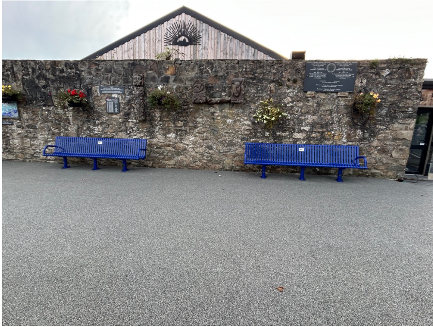
Image 3: New benches placed on the new surface
