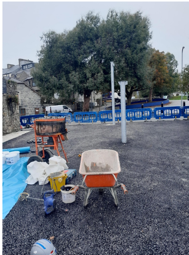
Image 2: New surface being installed after removing the old surface
